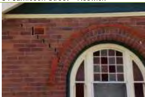
Detail of cracking on the front façade of 34 Jamieson Street - 'Keswick'.
