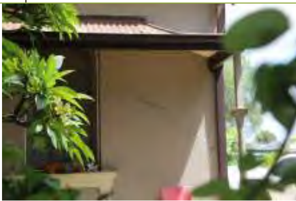
Detail of cracking to render on front façade.
