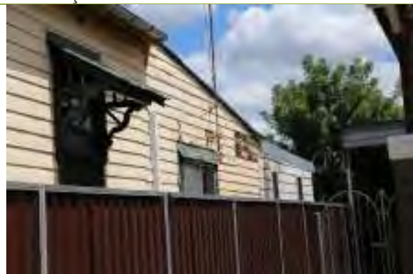
Detail of acrylic paint peeling and timber rot on the north elevation.
