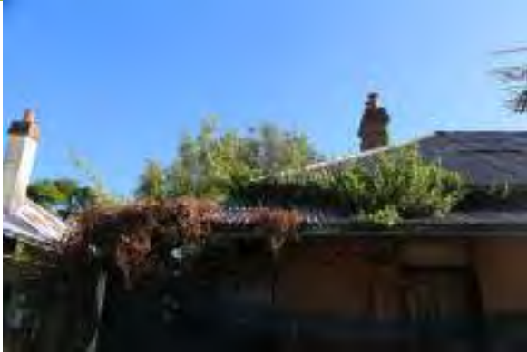
View of severe vegetation overgrown and impacting the verandah roof and guttering.
