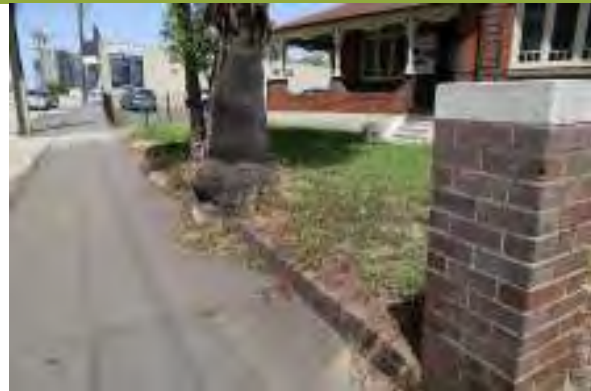
Removed fencing from the front elevation and large palm impacting brick retaining bed.
