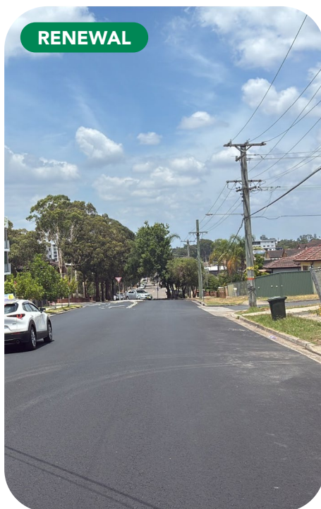
Windsor Road, Merrylands
