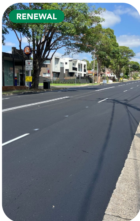
Merrylands Road, Merrylands
