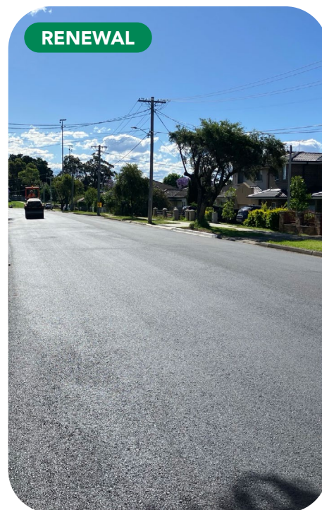
Major Road, Merrylands
