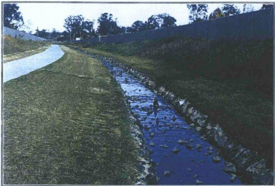
Plate 5 The rock lined concrete channel in Area III
