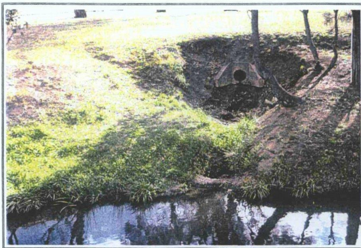
Plate 14 Stormwater outlets require rock lined flow dissipaters, siltation traps and trash racks, where appropriate
