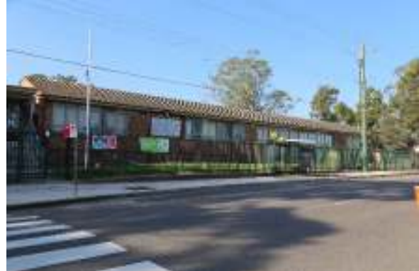
View of school from Ringrose Avenue.
