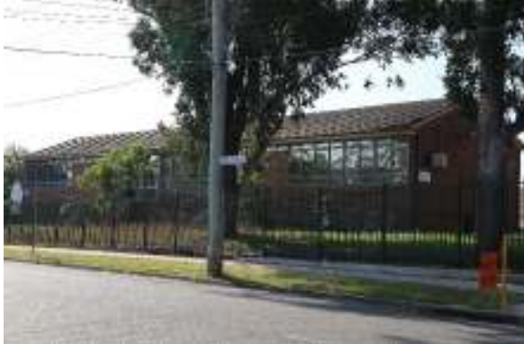
View of school from Ringrose Avenue.
