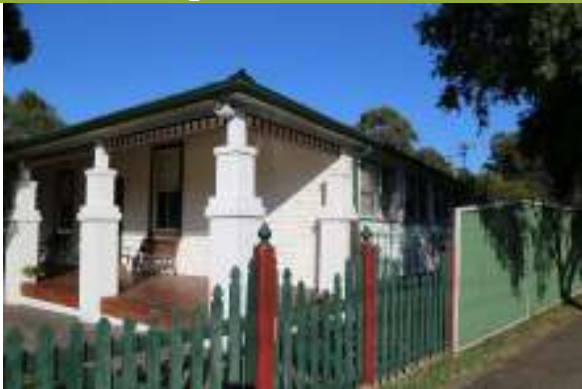
Detail of verandah.
