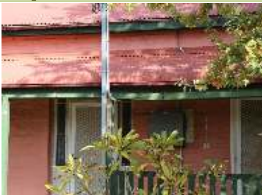
Detail of verandah and deterioration of timber.
