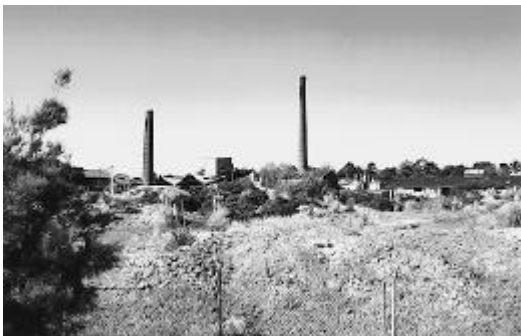
As the former brickworks site is redeveloped, access will need to be provided between this site and the park.
