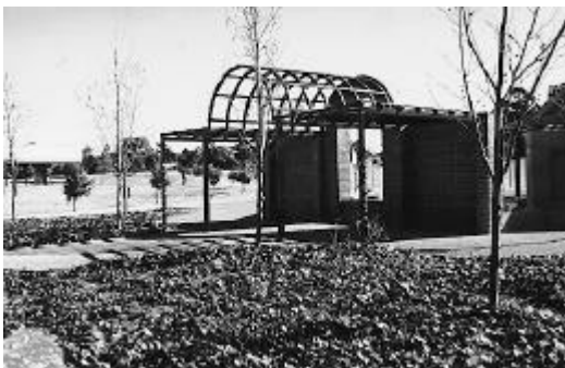
An number of commercial opportunities exist at Holroyd Gardens Park using existing infrastructure
