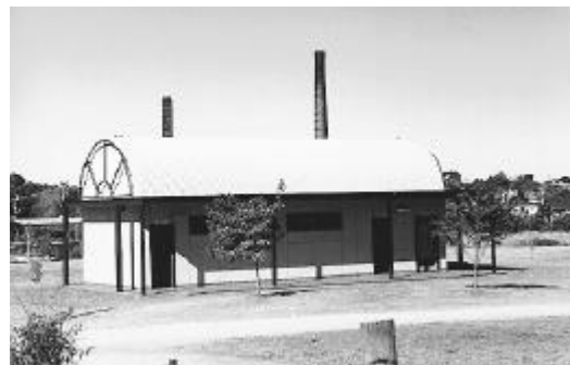
All buildings in the park are connected to water, sewage and electricity
