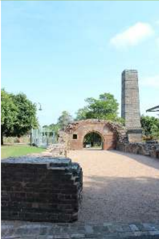
View to remnant structure and square-ended chimney.
