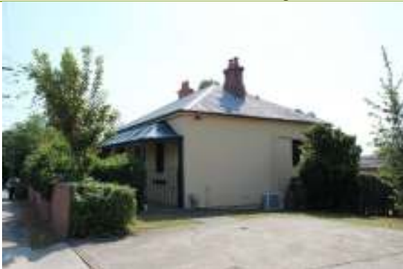
Western and southern elevations of Pitt Cottage.
