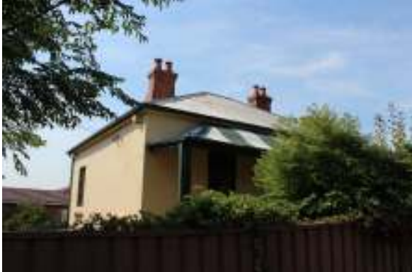
View to roof elements at Pitt Cottage.
