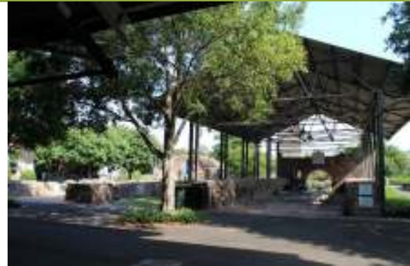
Overview of remnants of Goodlet and Smith Brickworks Site.
