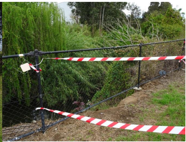
Erosion between sportsground and creek bank
