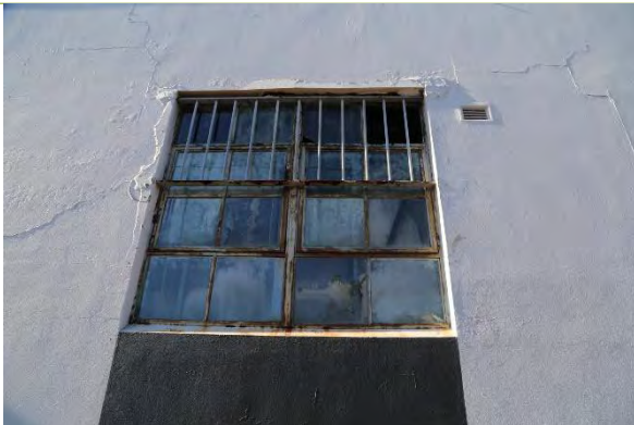
Detail of rusted window on elevation.
