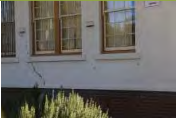
Detail of cracking to brickwork along front façade of main building.
