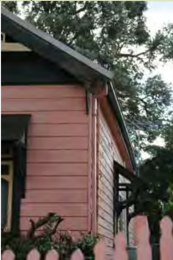
Detail of deteriorated timber to barge board.
