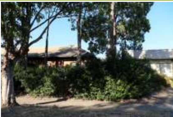
View from Arthur Street to Former Council Chambers showing 1970s extension.
