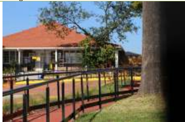
Detail of walkway and balustrade.
