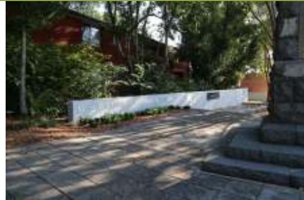
Rendered brick retaining wall with park name.
