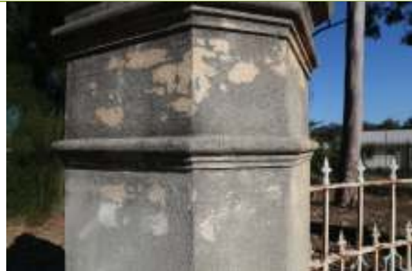
Detail of rendered post with painted coating.
