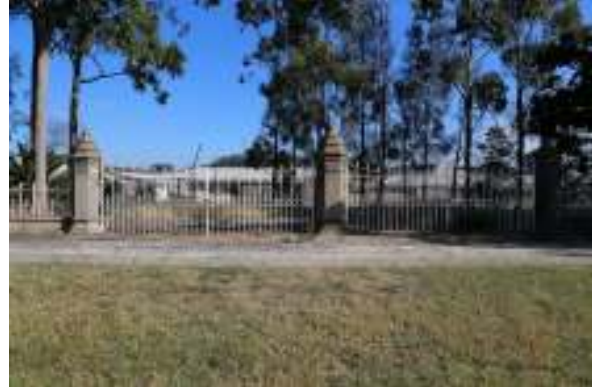
View west to Greystanes Gates from Greystanes Road.
