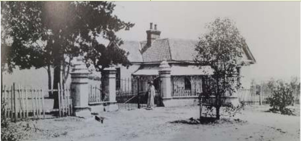
Greystanes Gatehouse and Gates, unknown date (Source: Historic Houses Trust, taken from Jane Ellias & Stephen Coppins, Pictorial History Holroyd , p.13).
