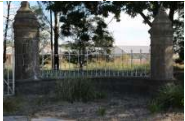
View of northern portion of Gates with replaced steel inserts.
