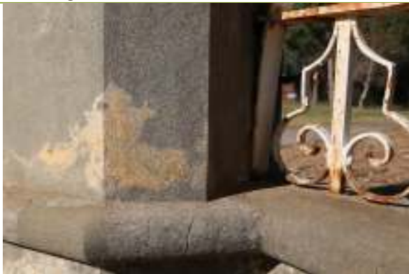
Detail of render and wrought iron post.
