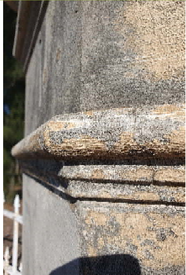
Detail of render and coating on post.
