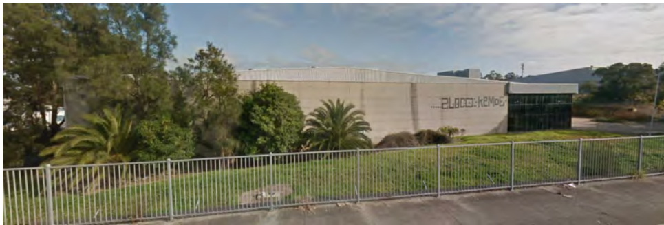
Figure 6 – Images of the Subject Site
