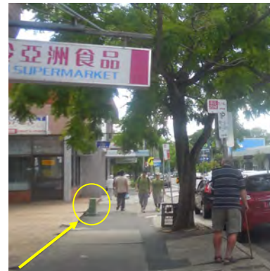
Uneven levels to be addressed, and small electricity box to be relocated to improve accessibility
