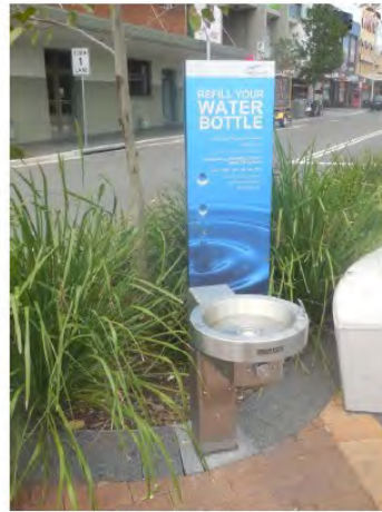
New Bubbler and water refill station.
