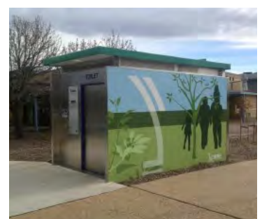
New public toilet with recyclable stainless steel and durable components, and efficient water usage
