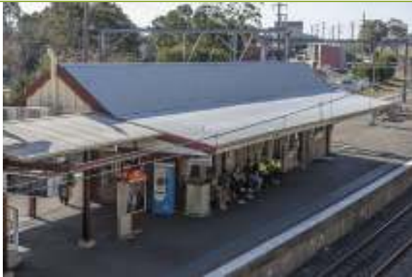
Platform building (Source: NSW Office of Environment and Heritage, Railcorp S170 Listing Sheet for Regents Park Railway Station Group).
