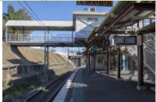
Footbridge (Source: NSW Office of Environment and Heritage, Railcorp S170 Listing Sheet for Regents Park Railway Station Group).
