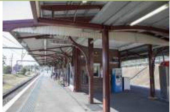
Underside of platform canopy (Source: NSW Office of Environment and Heritage, Railcorp S170 Listing Sheet for Regents Park Railway Station Group).
