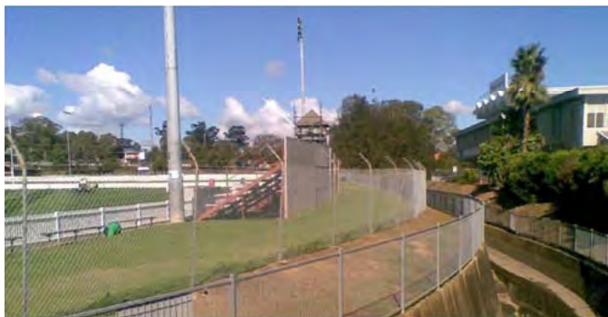
Photograph of existing structures
