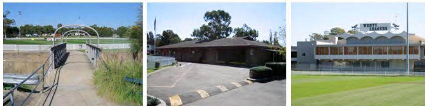
L to R: View across bridge towards Ringrose Oval from the carpark in the northwest corner, "the complex" facilities building at the northern end of Ringrose Oval, the Wentworthville Leagues Club from Ringrose Oval
