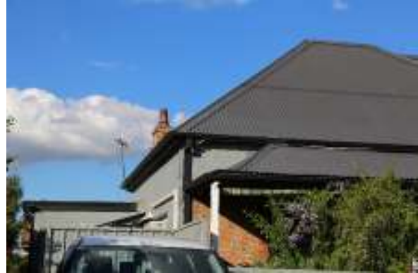
View of roof detail.
