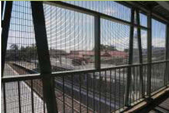
View northeast from concourse to Platform 1/2.
