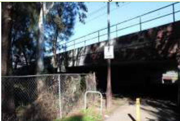
View from eastern edge of underbridge looking west.
