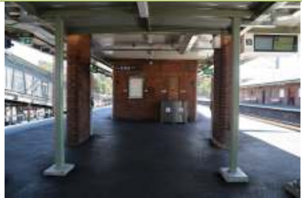
View north to Station Building on Platform 3/4.
