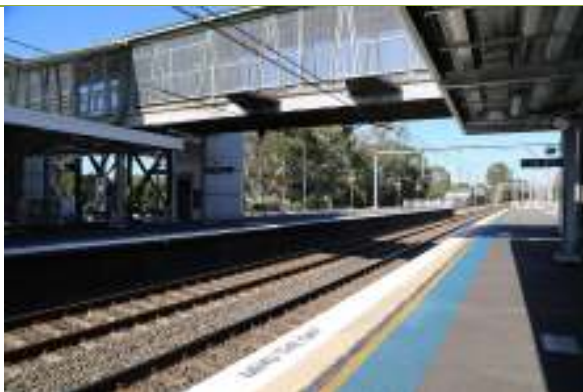
View southeast to Platform 2.
