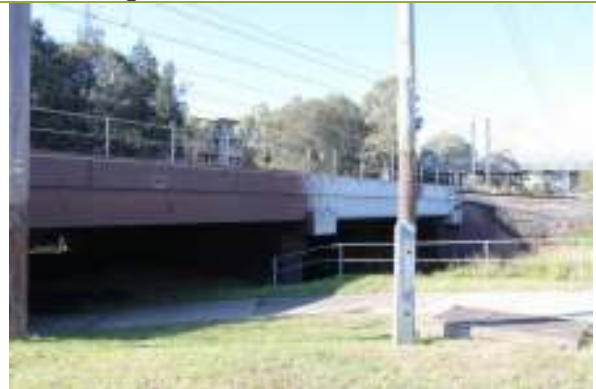
View east to Underbridge from Portico Parade
