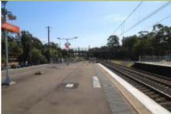
View north towards underbridge.
