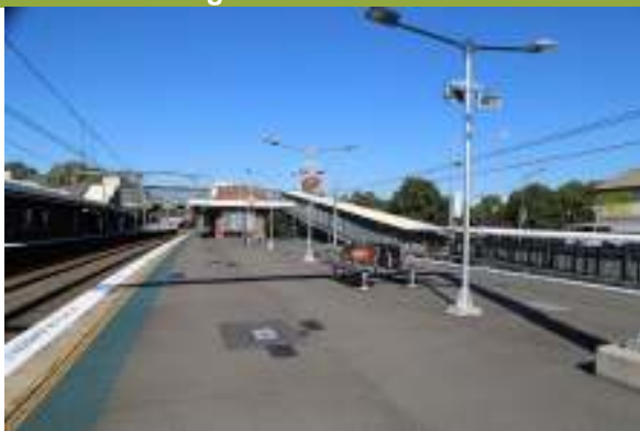
View south from platform towards concourse.
