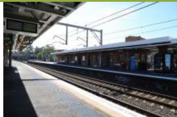
View from platform 3 to platform 2.
