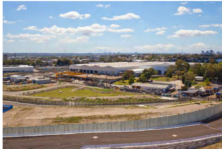
1. VIEW OF THE CLYDE MARSHALLING YARDS
