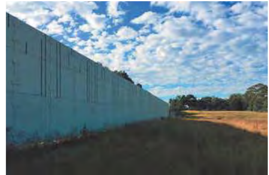
2. VIEW OF THE WALL CROSSING THE SITE
