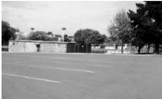
The carpark at the northern boundary of the Swimming Centre provides parking for all park users as well as access to the Wentworthville Youth Centre.
