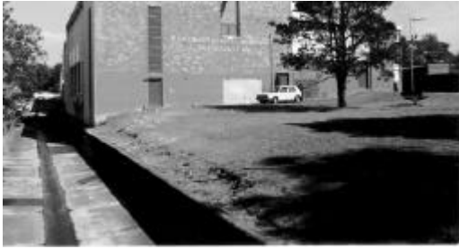
The Wentworthville RSL Club building, located on the boundaries of the south east corner of the park is visible in the background while the concrete drainage channel can be seen in the foreground.
