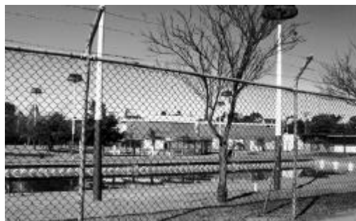
At present the Wentworthville Memorial Swimming Centre can only be used during summer months
