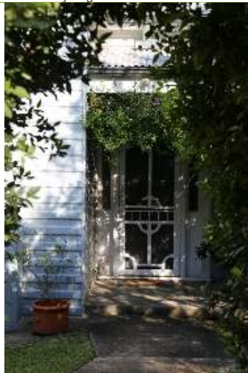
Detail of front door and rusticated weatherboards.
