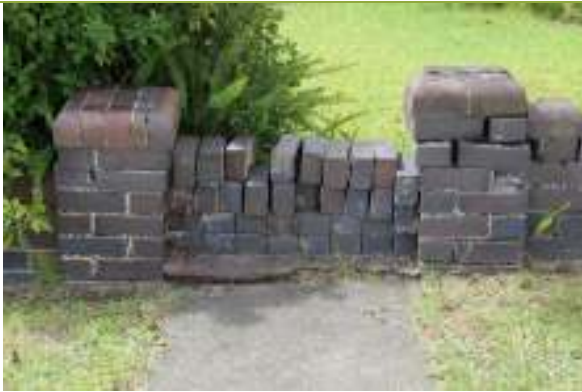
Detail of brick boundary fence in a poor condition.
