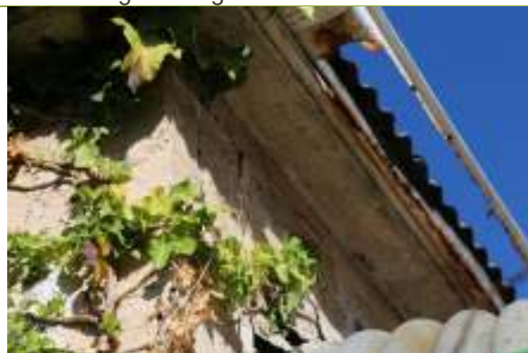
Corroded gutter the north elevation of the roof.
