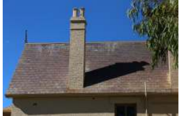
Detail of slate roof from Hawkesbury Road
