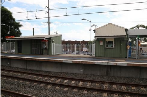
View to Platform 1 station elements
