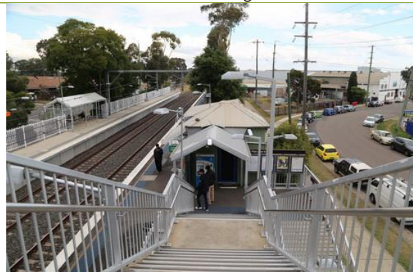
View northeast from Footbridge to Platform 1.
