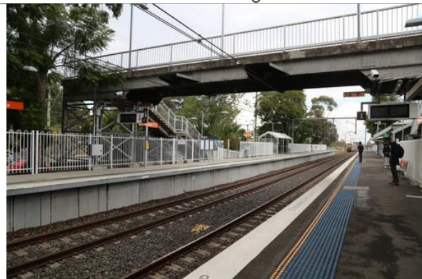
View of footbridge from Platform 2.
