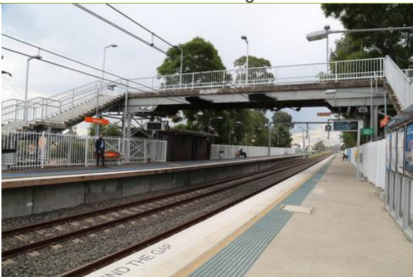
View from Platform 2 southeast to Platform 1.
